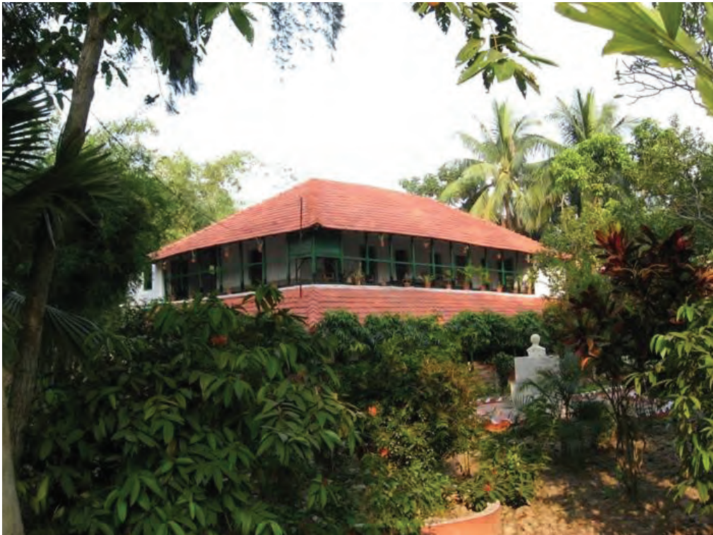
Sarat Chandra's Habitat at Samtaber, after restoration.
